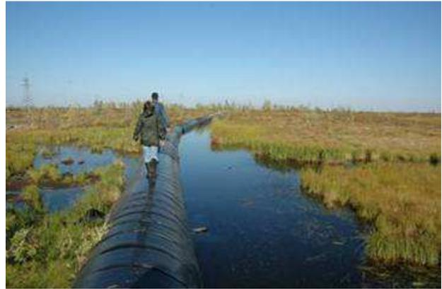
b) Floating pipeline initially buried in fill
