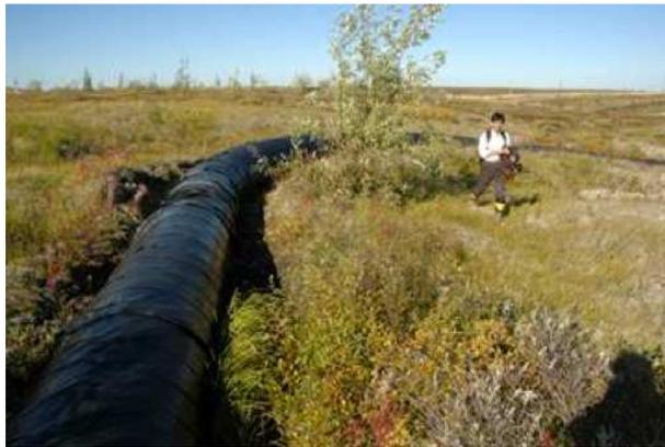
c) Exposed pipeline initially buried in fill
