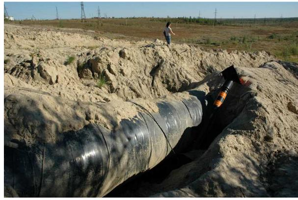
d) Exposed pipeline in a slope
