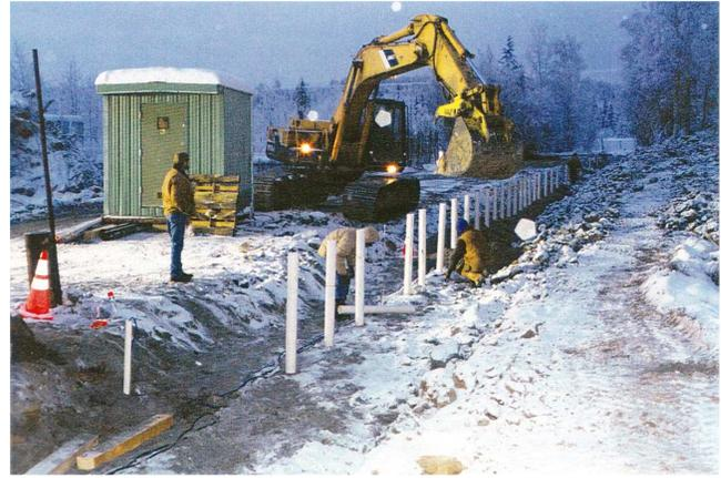
b) Plastic casings enclosing heave rods
