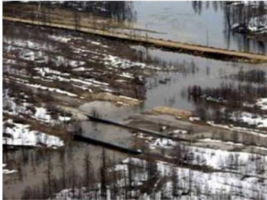
a) Washed and exposed pipelines
