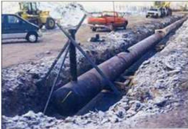
c) Welded test gas pipeline right before the lowering
